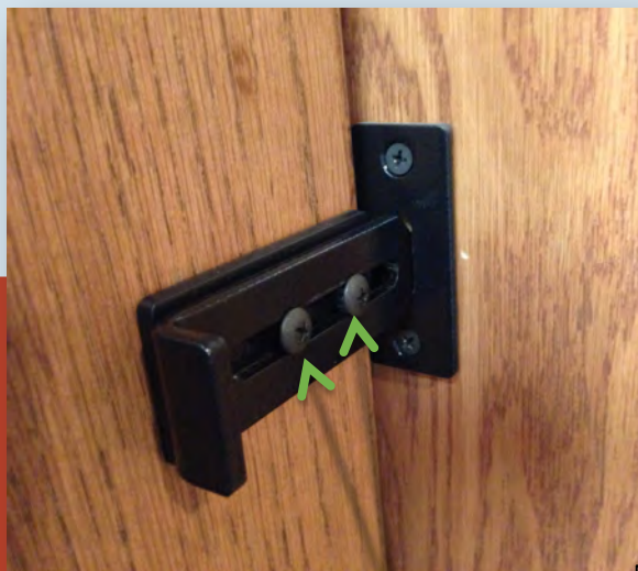
Tighten Screws to Desired Tension
